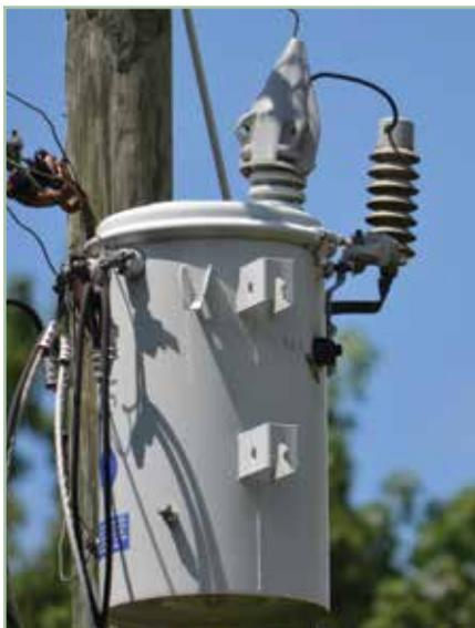
*The top image shows a fused cutout. The fuse will blow when a fault occurs on the line. The bottom image shows a squirrel guard (cone-shaped) over the high side bushing of the transformer. This helps prevent outages caused by small animals or birds.*
