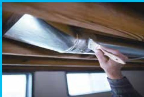
*Your ductwork should be sealed with mastic at all connections and seams to ensure conditioned air leakage is kept to a minimum.*
